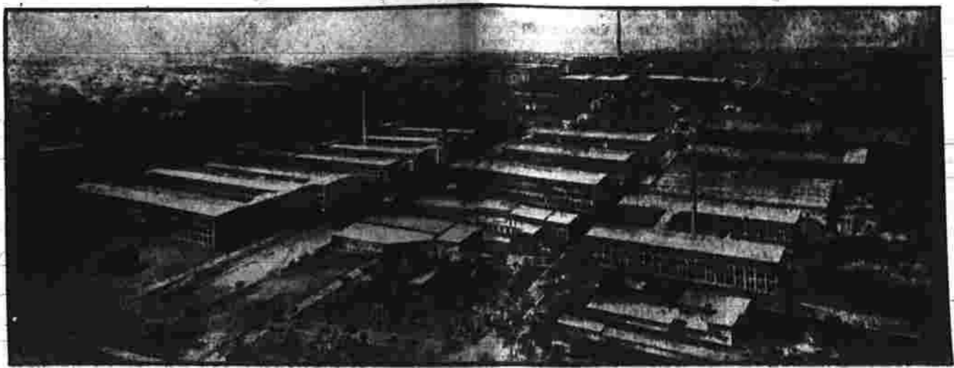
The March of Progress Panorama of the Present Plant
